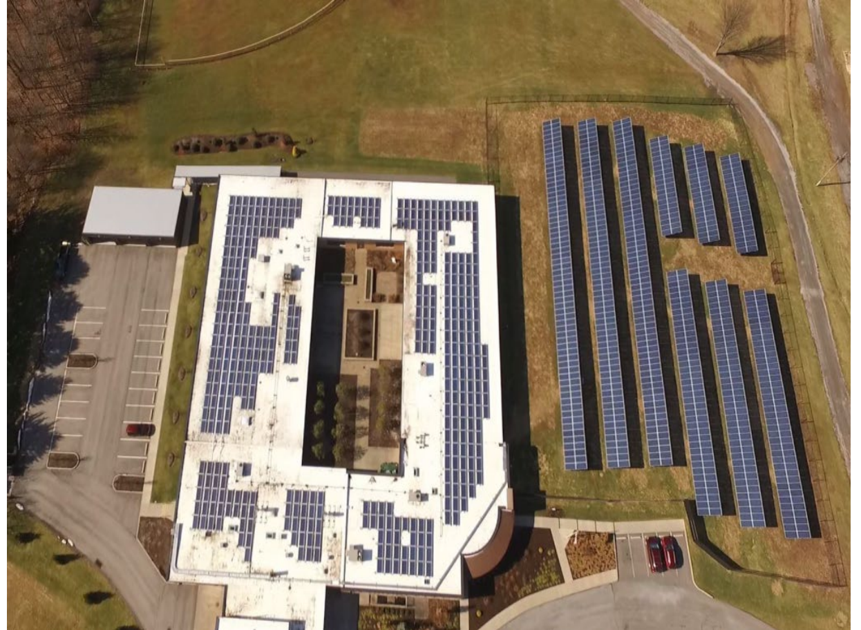
The 365kW system at the Felician Sisters of North America Headquarters in Beaver County, Pennsylvania.
